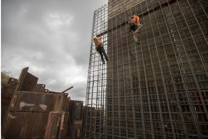
Workers tie rebar on a support structure as construction continues in Fresno on the California high-speed rail project. (Robert Gauthier / Los Angeles Times)
